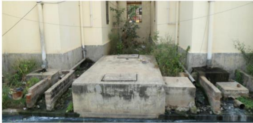
Stagnated water from the septic tanks at the back lanes of the blocks at Lambert Saravanan Nagar site
